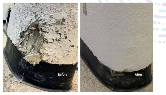
• Repair of damaged column due to smart-carts, golf carts and other luggage on the second floor of MIA's Central Terminal by Door No. 17.
