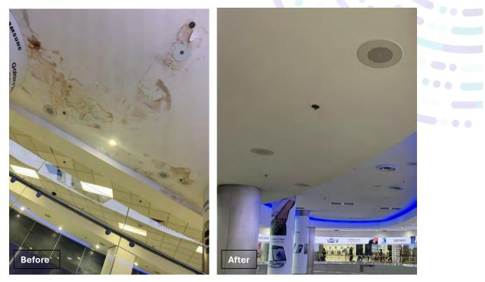
• Repair of the tear drop ceiling areas caused by roof leaks on the second floor of MIA's North Terminal by Door No. 8.
